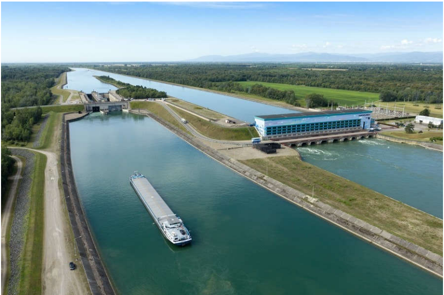
The hydroelectric power plant installed on the Grand Canal d'Alsace product annually on average about one billion kWh.
