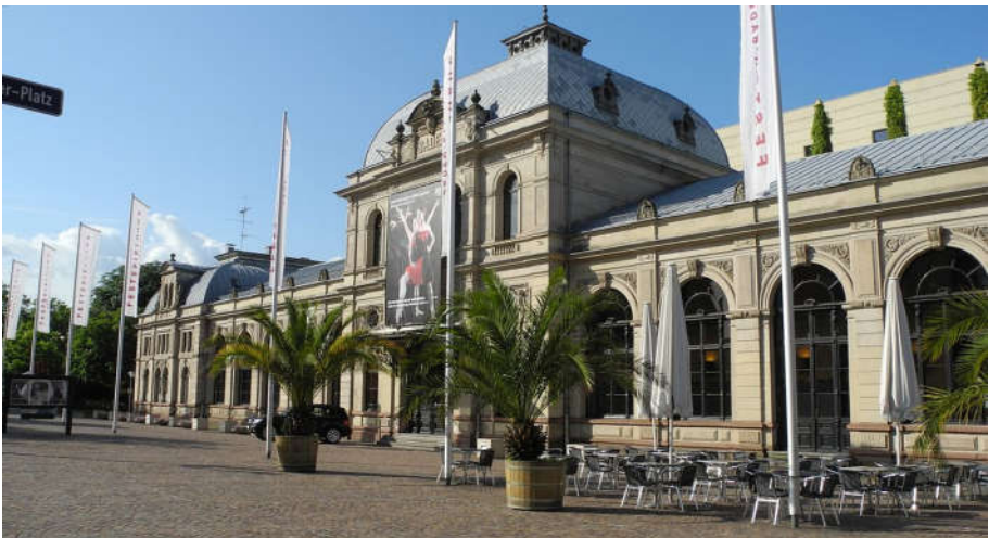
The old station Neo-Renaissance style with Baroque elements, is the input of the Festspielhaus - a very modern building.
